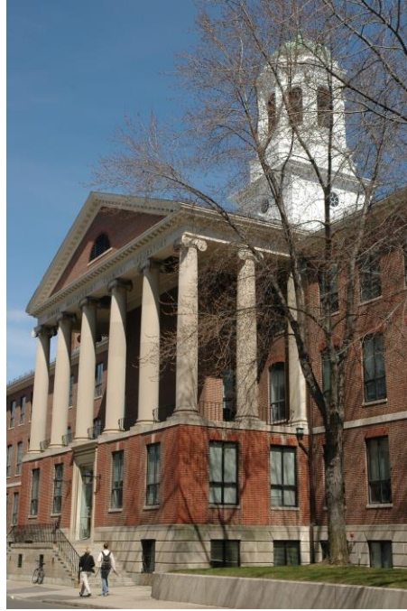
Mallinckrodt Building (Chemistry)
